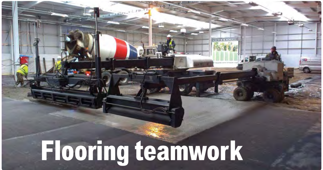
Somero SXP laser screed and STS topping spreader in action.
